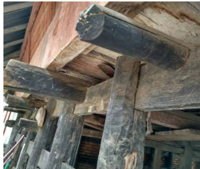
Figure 7. Building floor supported by the wooden blocks
